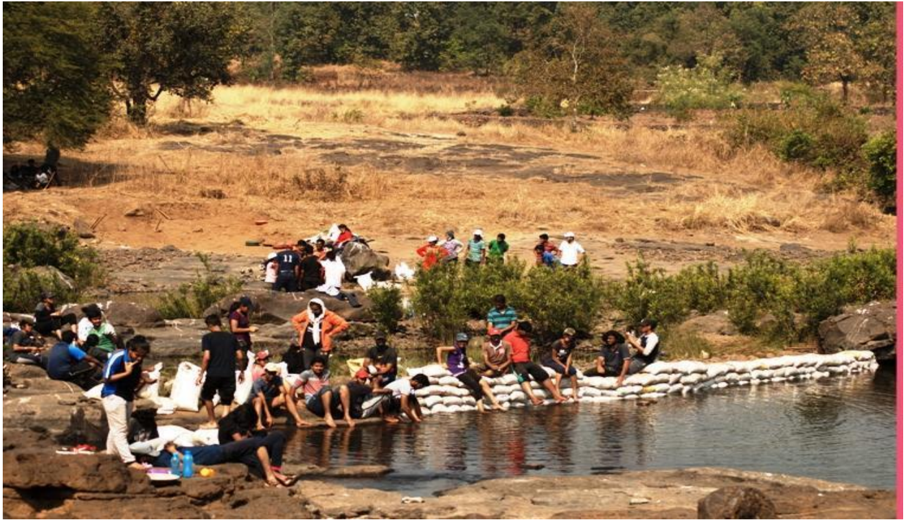
WORKING ON DAM 1
